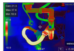
Hot water pipes verification
