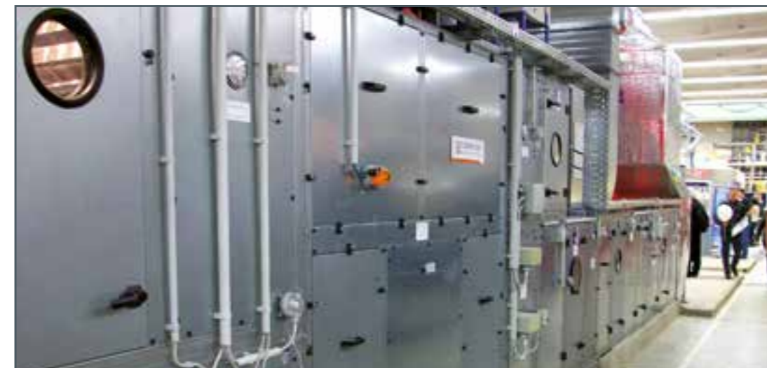
Direct evaporator as air cooler
