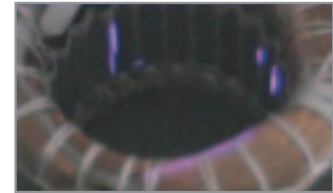
Figure 8: Corona discharge in motor
